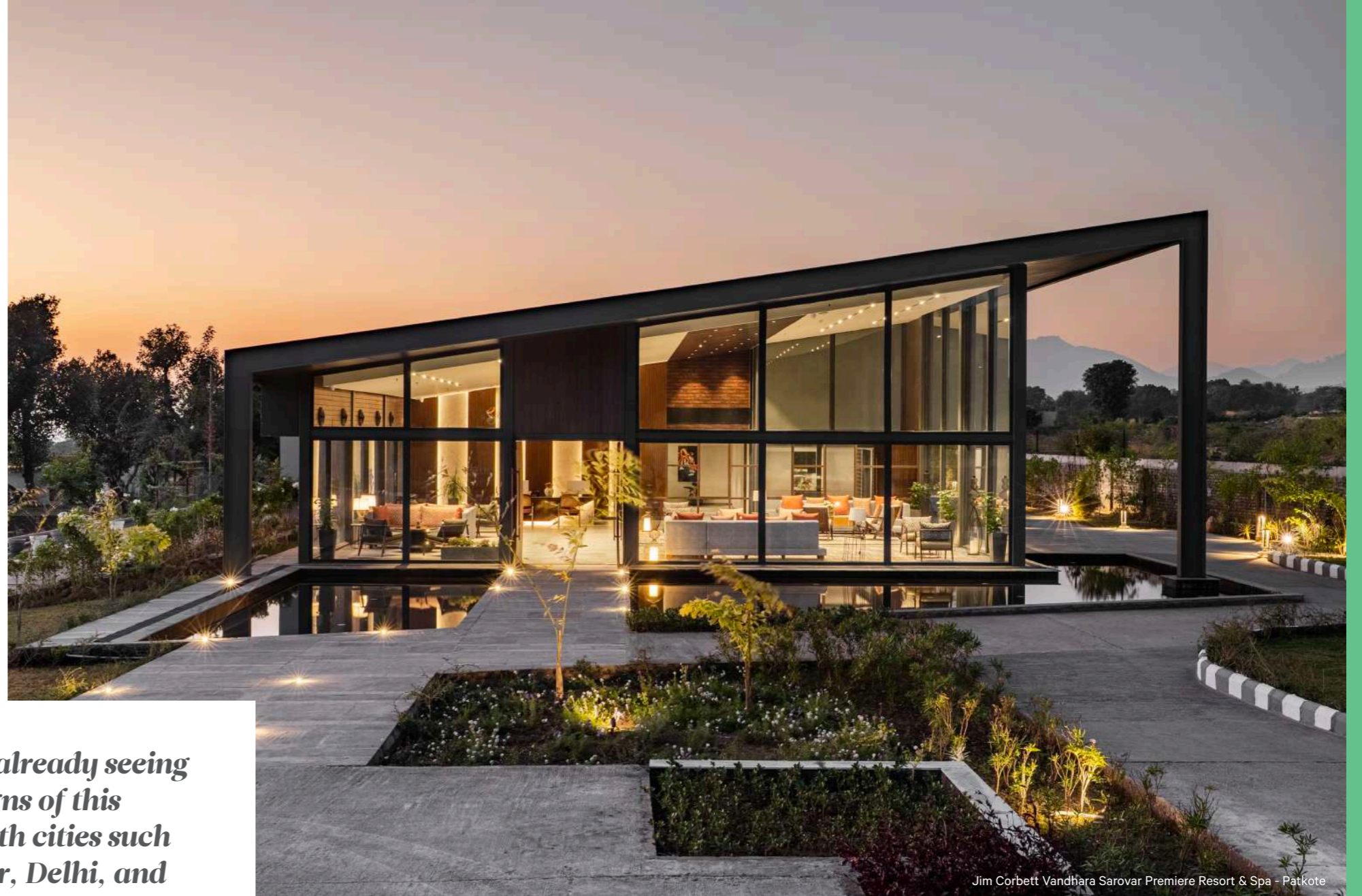
Hilton Garden Inn Mumbai International Airport
